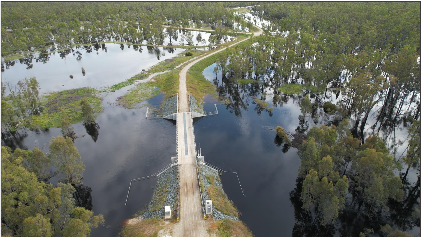
Figure 5: View north over Barbers Ck regulator to Cow Ck regulator top centre, Moulamein/Barham Road top left to centre and Koondrook Forest to the right.
