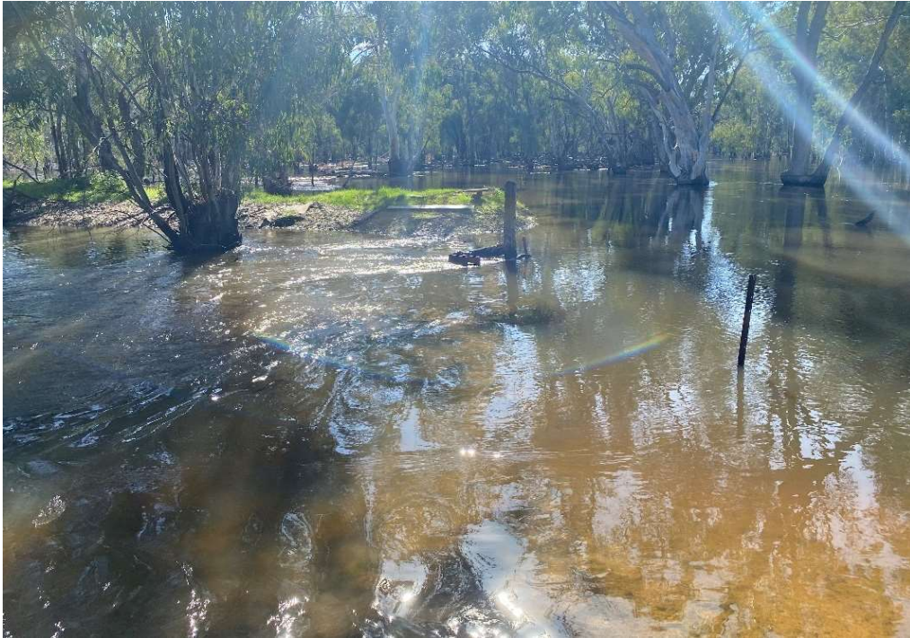
Figure 11. Location of the Sheep Wash Lagoon regulator at the Merran Creek offtake into the Sheep Wash Cutting – structure overtopped at time of site inspection due to high flows (31,000 ML/d at Torrumbary Weir on 9/08/2023).
