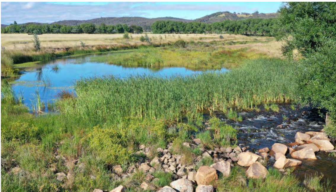
Figure 18. Example of an established in-stream 'leaky weir' structure on the Mulloon Creek.
