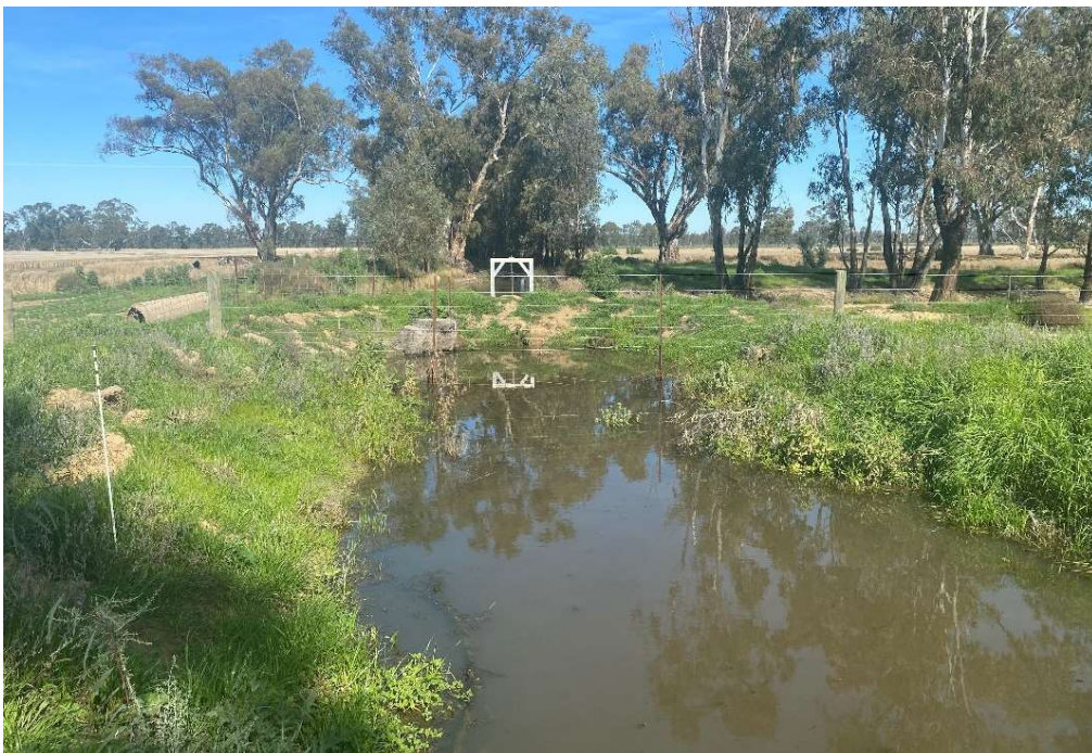
Figure 12. Irrigation channel with control gate on Gonn Station which could potentially be utilised for the delivery of environmental water to Sheep Wash Lagoon.
